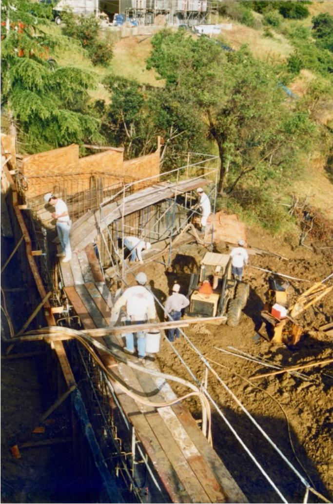
beam structure of the entire wall and applied an 8 inch thick layer of sprayed concrete. We also attached a 1 inch diameter metal rebar structure along the entire top of the wall and had the entire unit coated with shotcrete.
